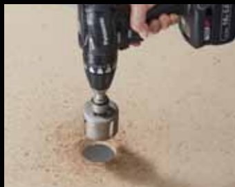
Drill vertically into boards
