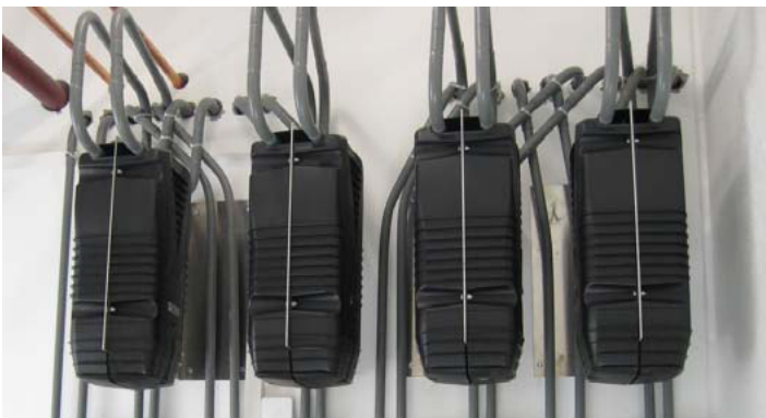
Vulcans installed back to back.
