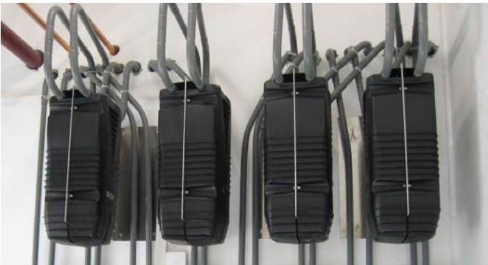
Vulcans installed back to back.
